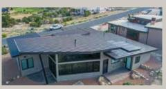
Snap-Lock 1.5" Roofing is at its best when it is applied in a Direct to Deck fashion. Using a furring strip could cause the panels to unsnap if stepped on.
